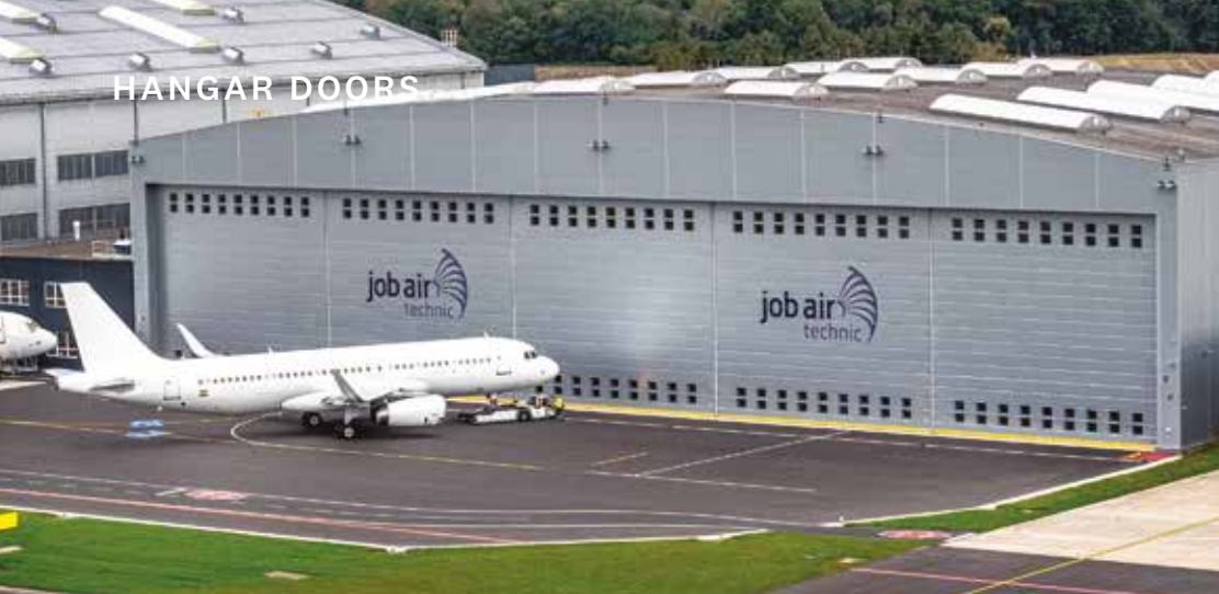
◀ Champion Door created a large hangar door for Job Air Technic at Ostrava-Mošnov airport
